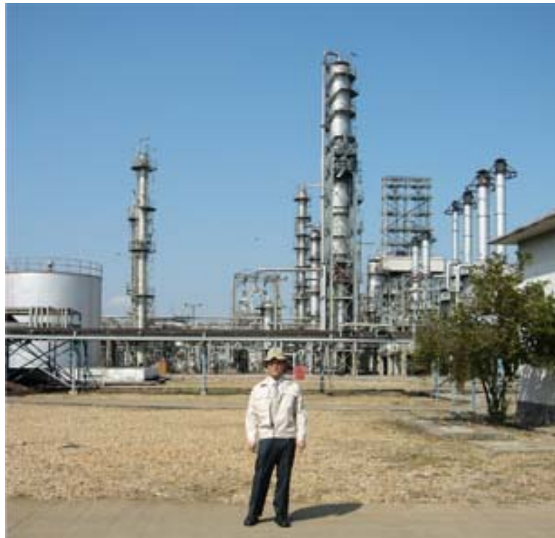
Photo -3-1 Refinery Tower of Thanbayakan Oil Refinery (Atmospheric Distillation Plant, etc.)
